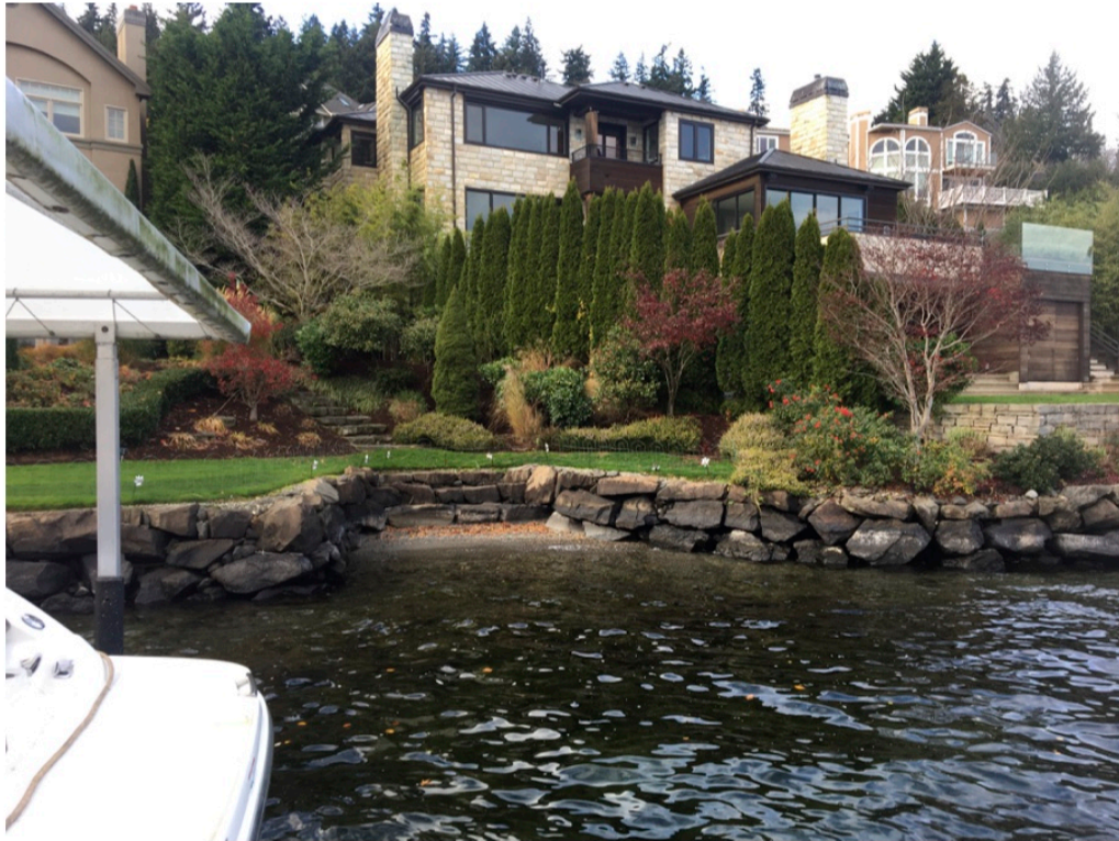
Photo 3 - Existing cove in shoreline
